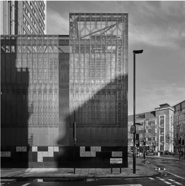
Bunhill Energy Centre utilises warm air created by machinery and trains on the London Underground for district heating.
